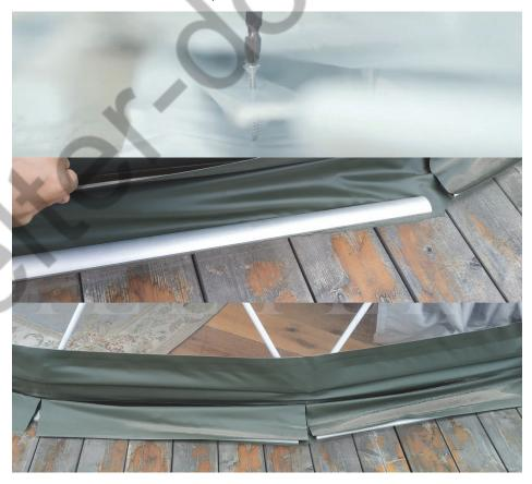
[Step 2]: Use bolt "M6\*25" to secure the aluminium strips on the door frame (up, left and right entrance units), cover with related aluminium caps.
